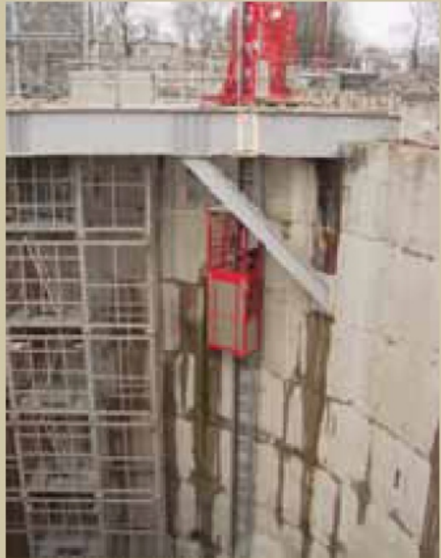
This Stros BV 400 hoist has 400 kg of lift capacity.
